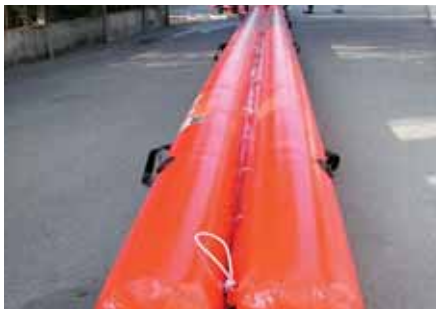
Ambos tubos deben apretarse antes de recibir el monotubo Tubes must be well tightened before receiving the monotube
