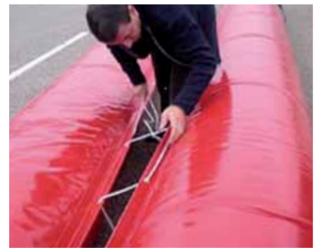
Atadura de 2 Tubos Lacing the two tubes
